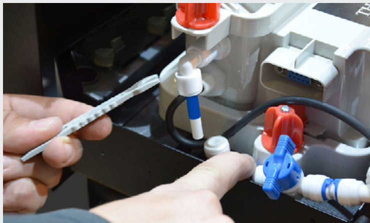
12 The piping unit inlet is now separated from the sump.
